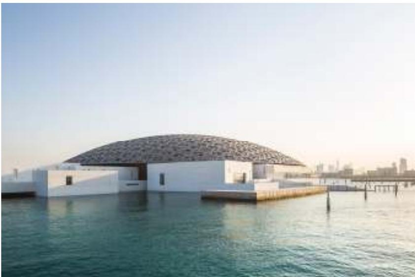
The centrepiece of the museum is a huge silver dome that appears to float above the entire museum. In fact it weighs 7,500 tonnes (the same as the Eiffel Tower in Paris). The dome is a complex, geometric structure of 7,850 stars, repeated at various sizes and angles in eight different layers. As the sun passes above its light filters through the perforations in the dome creating a 'rain of light'. This was inspired by the way light passes through the palm trees and filters through to the ground.
